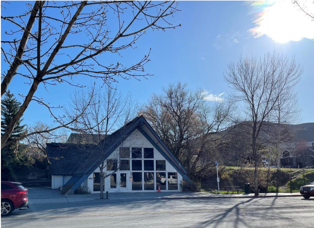
1. Front of Building
