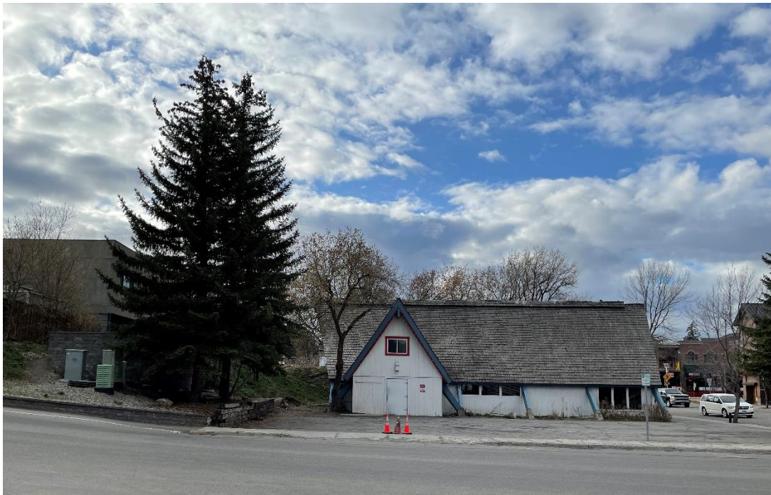
2. Side of Building
