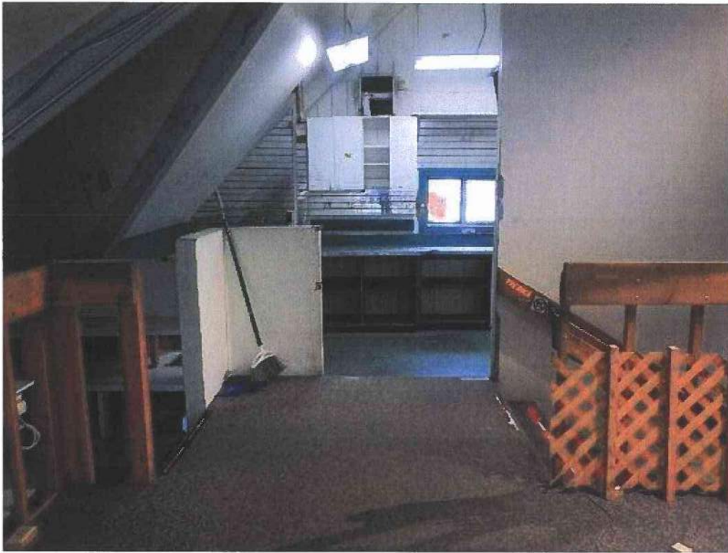
Photo 23: Work room on mezzanine level Note: sheet vinyl floor, fan and exhaust piping
