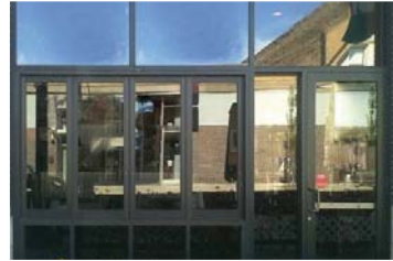
EXTERIOR DOORS AND WINDOWS: BLACK ANODIZED STOREFRONT
