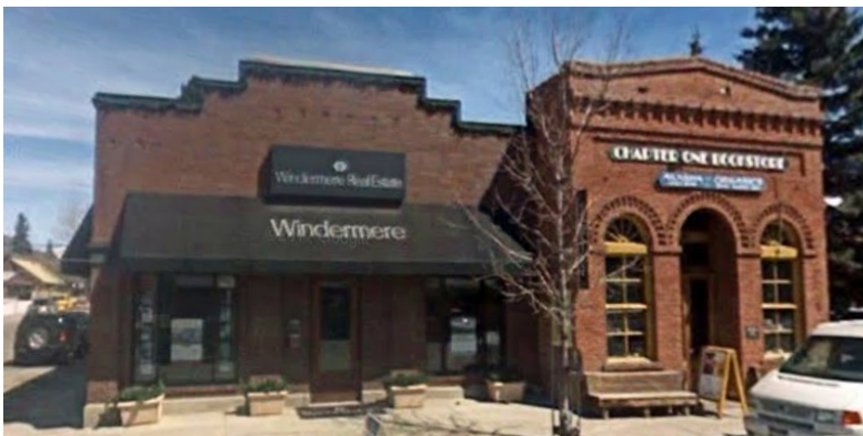
Before apartments added
