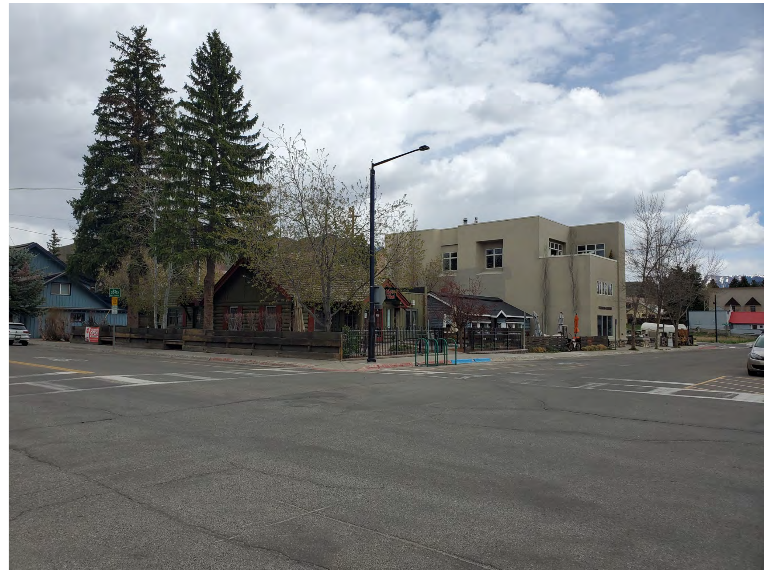
VIEW LOOKING EAST
