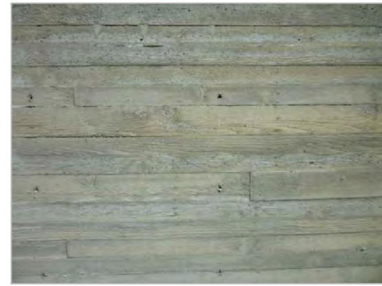
CONCRETE SITE WALLS
