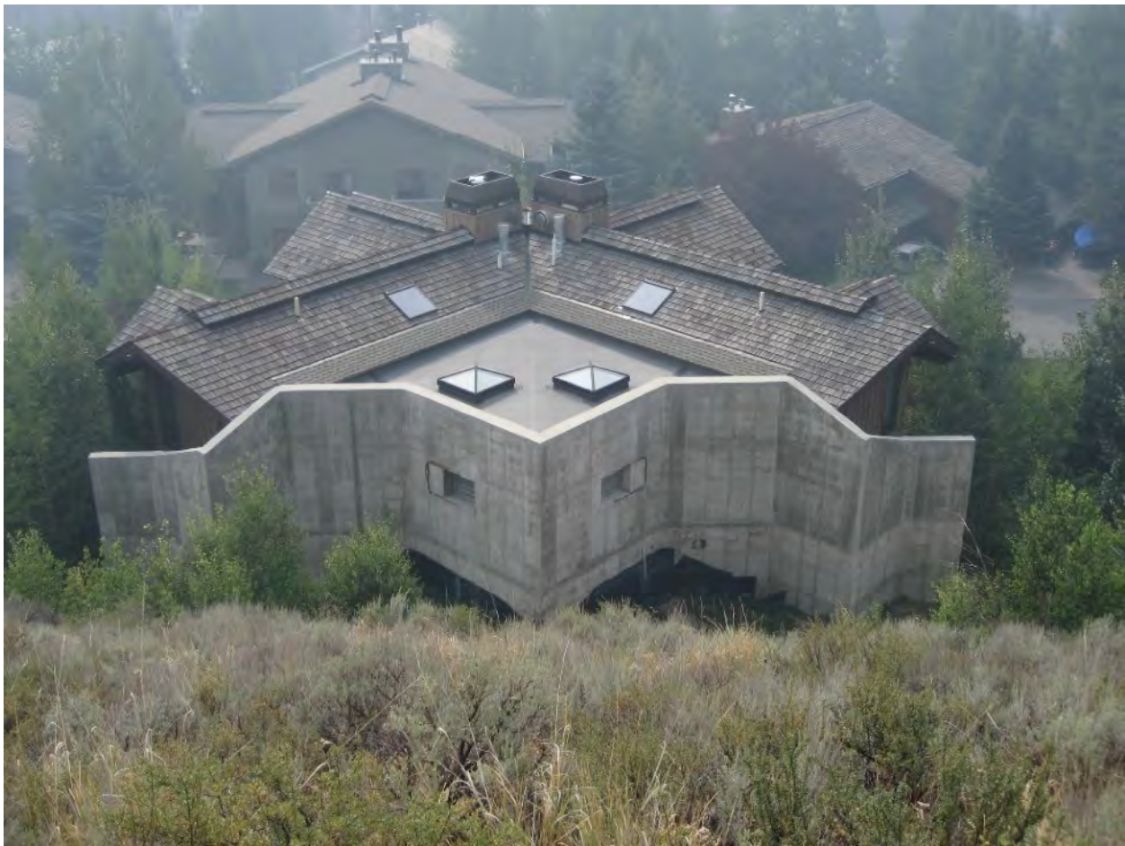
392 & 394 Sage Rd Avalanche wall integrated with building. Sits on massive footing with 2' deep keyway extending below footing to resist forward displacement.
