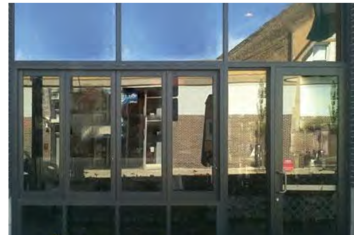
EXTERIOR DOORS AND WINDOWS: BLACK ANODIZED STOREFRONT
