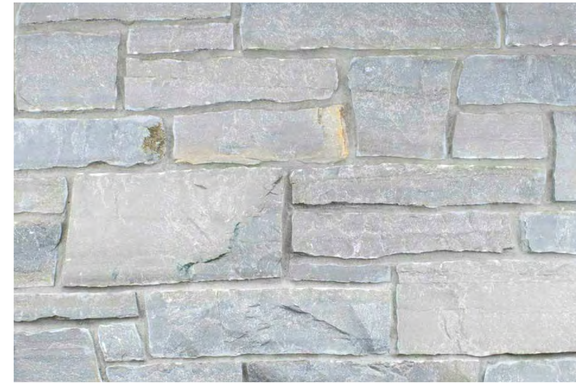
EXTERIOR FINISH 5 (EF-5): NATURAL STONE VENEER ASHLAR PATTERN, COLOR:
