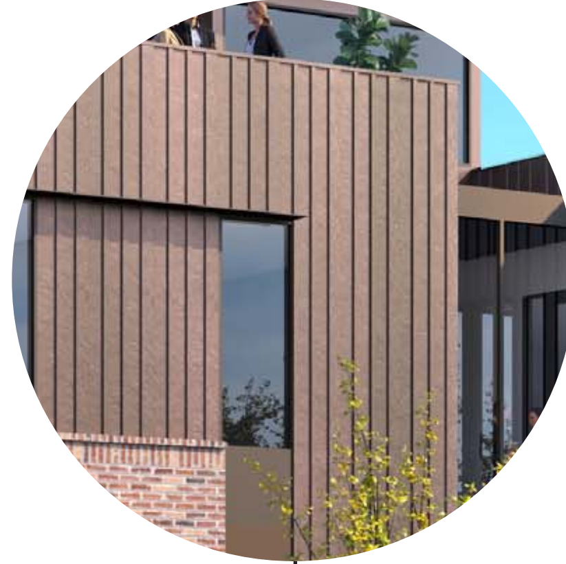
BONDERIZED VARIABLE WIDTH VERTICAL BOX SEAM METAL SIDING (PERFORATED AT SCREENS)
