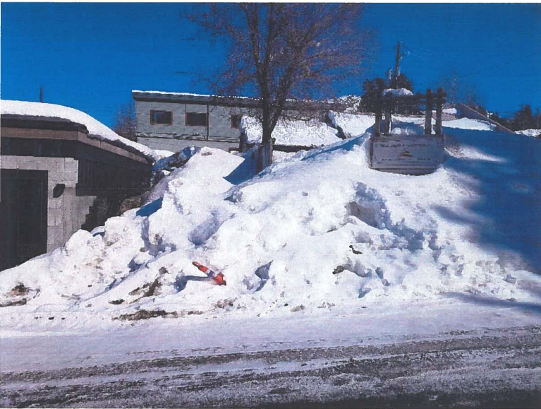
2 - Existing Site Conditions - Lot 3 existing grade at base of wooden sign. Grade in between sing and building is 3' lower than pavers.
