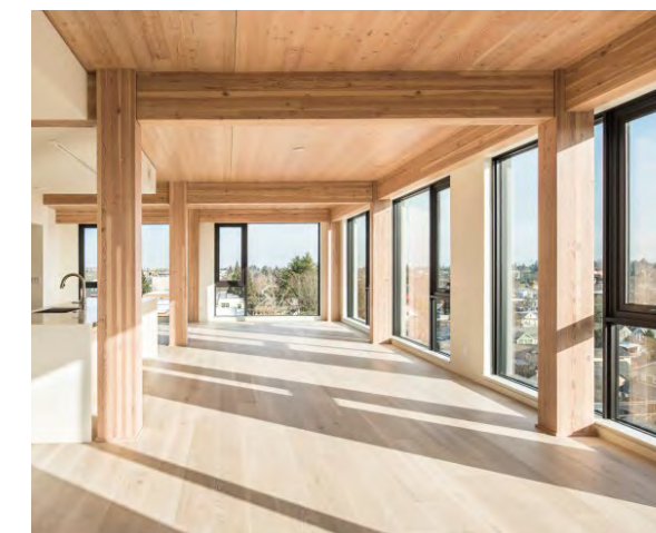
CLT Structure Smartlam, Montana
