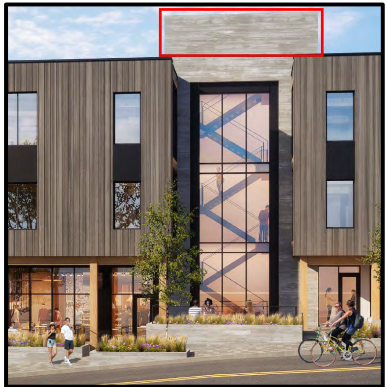
Figure 4: Stairwell & Elevator Shaft Extending Above Roof Surface
