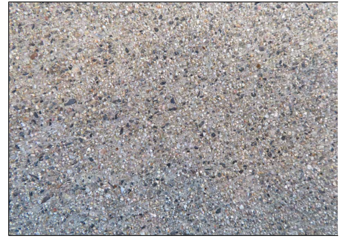
EXTERIOR FINISH 7 (EF-7): EXTERIOR CAST-IN-PLACE CONCRETE SLAB; ACID ETCHED CONCRETE WITH LIGHTLY EXPOSED AGGREGATE
