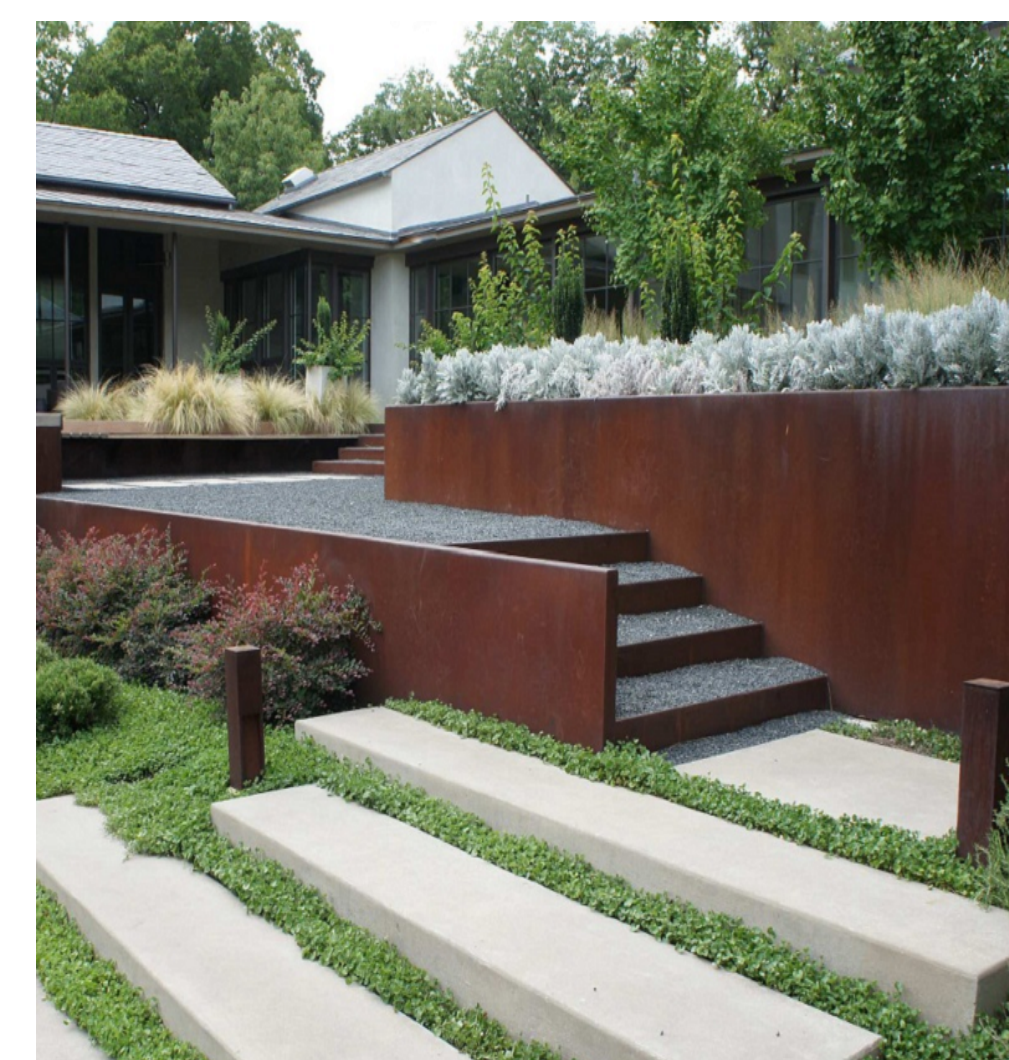
CONCRETE W/ STEEL PLANTERS AS RETAINING WALLS
