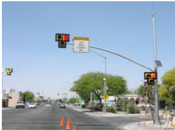
STC optically-activated fire station warning signal
