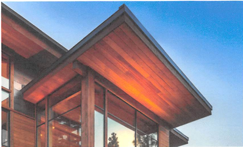
Soffit- 1x4 Cedar Shiplap To Match Siding
