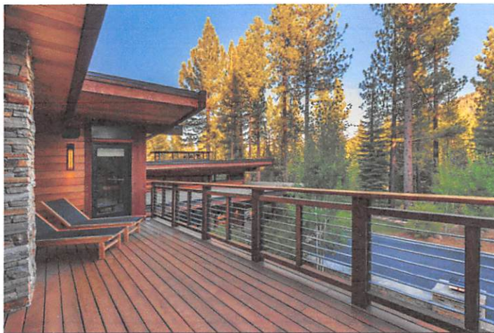
Metal and Wood 2 nd floor patio railing
