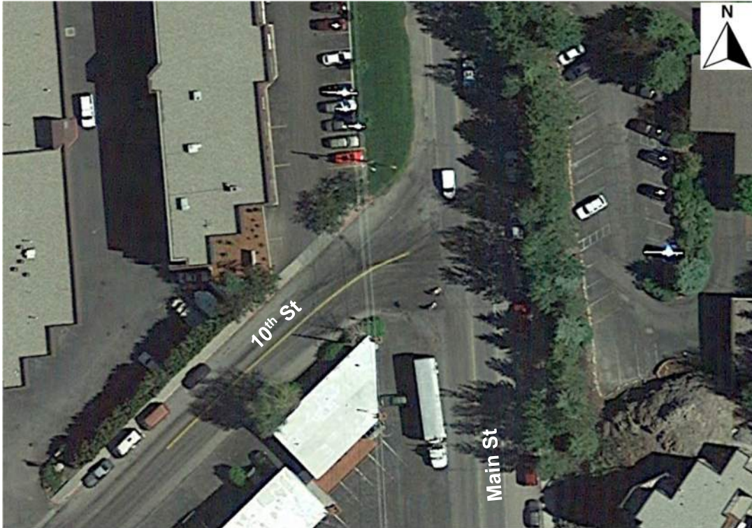
Figure 6. 10th Street and Main Street (SH-75) Intersection Area
