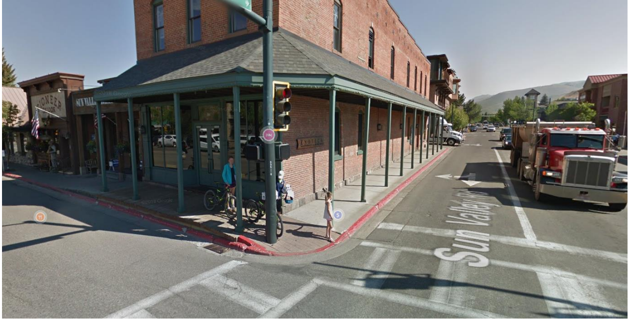
Figure 11. ADA/PROWAG Noncompliant Corner at Sun Valley Road and Main Street
