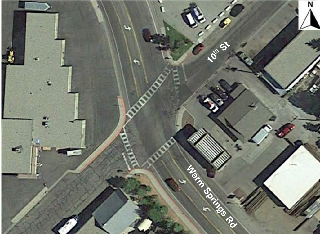
Figure 5. 10th Street and Warm Springs Road Intersection Area
