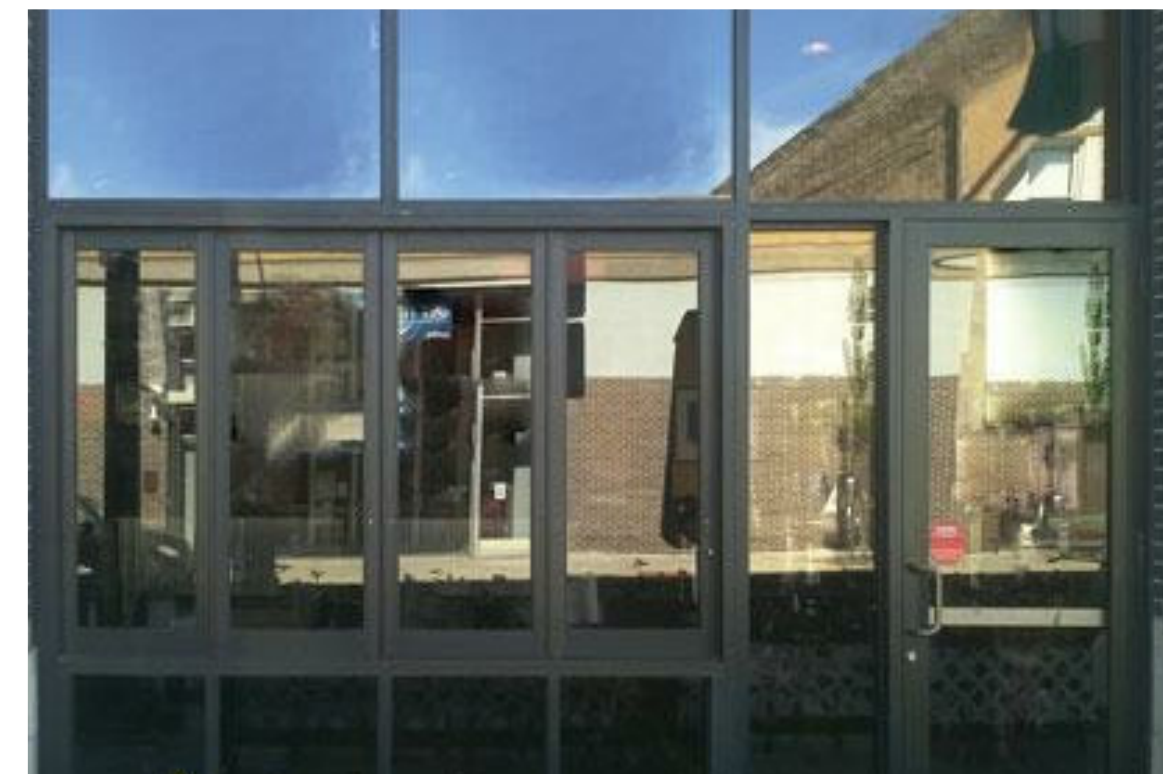
EXTERIOR DOORS AND WINDOWS: BLACK ANODIZED STOREFRONT
