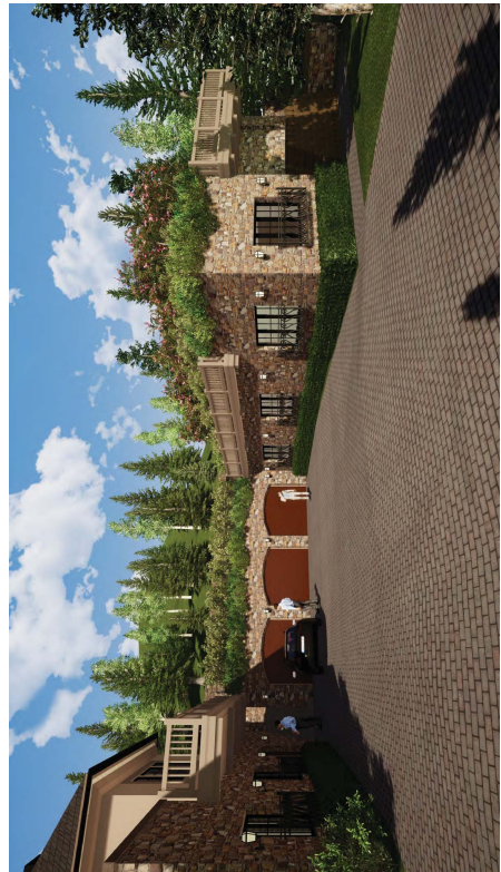
VIEW LOOKING NORTHEAST TOWARDS ADDITION
