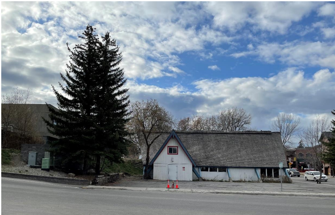
2. Side of Building
