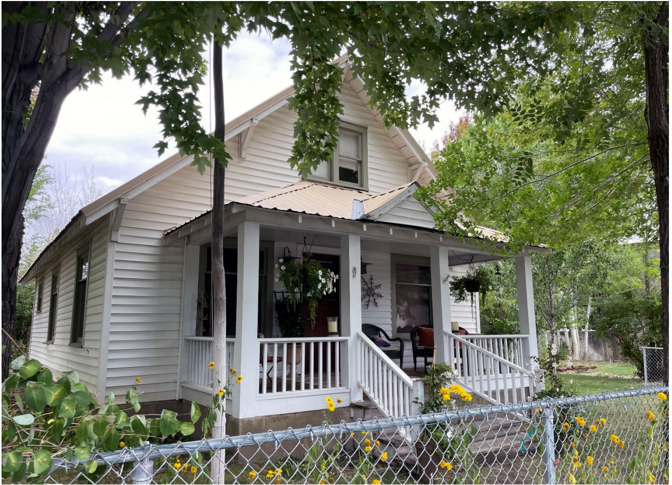
Photo A: Front Porch, Northwest side
