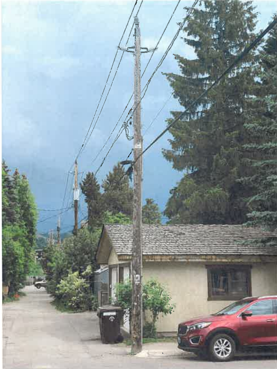
VIEW LOOKING SOUTHEAST FROM 8 TH STREET
