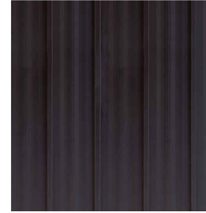
STANDING SEAM ROOF
