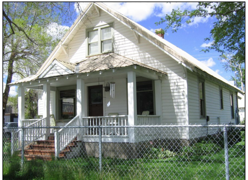
Figure 2: Existing Historic Home at 180 N Leadville
