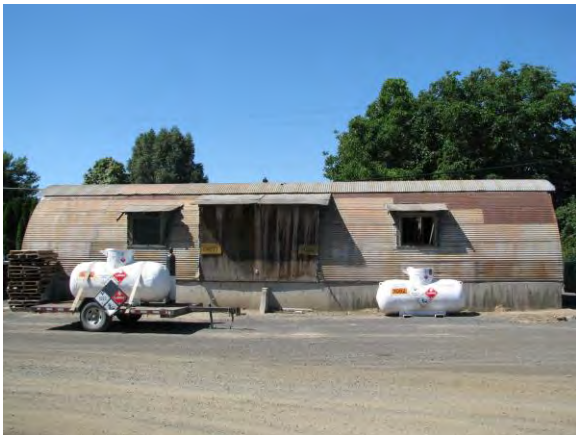
Note entrance in center that was removed and plywood placed over it. Reclamation digital photo by Kelsey Doncaster. 6/5/2015. Building No. 1423 front elevation. 2015
