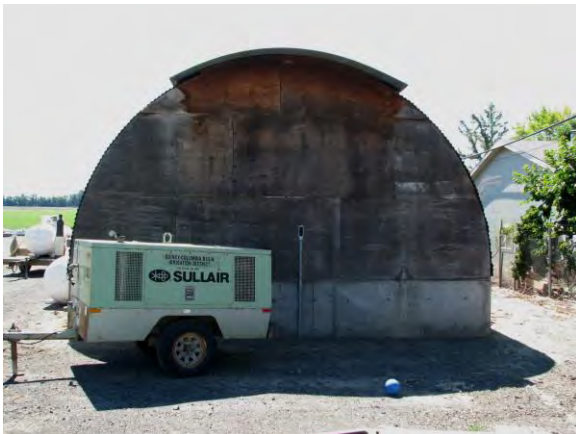
Note the solid plywood wall where windows and clapboard had been. Reclamation digital photo by Kelsey Doncaster. 6/5/2015. Building No. 1423 looking southeast at northwest elevation. 2015
