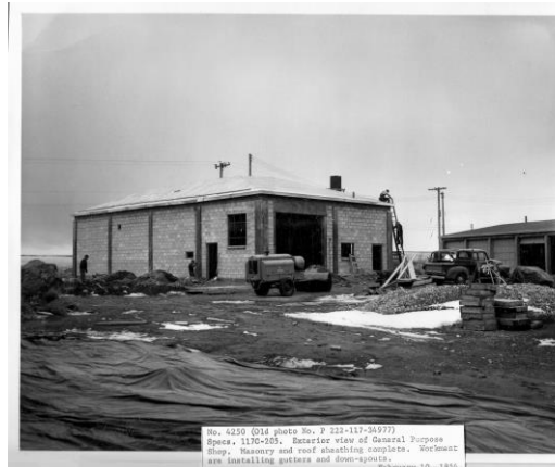
Exterior view of General Purpose Shop. Masonry and roof sheathing complete. Workmen are installing gutters and down-spouts. Reclamation photo No. 4250 taken on February 10, 1954. Royal General Purpose Shop under construction. 1954
