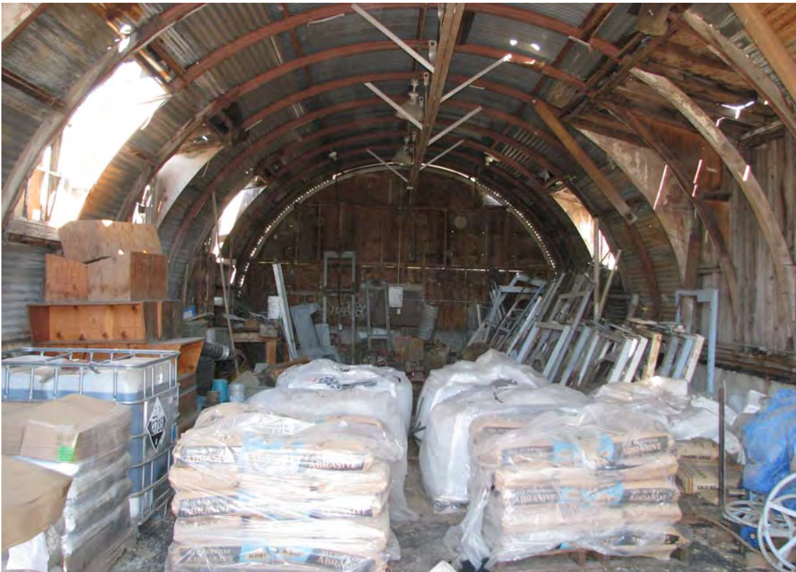
Figure 9: Building No. 1423 interior looking northwest. Note the interior walls are all gone and a trolley rail had been installed at the top. June 5, 2015. Reclamation digital photo by Kelsey Doncaster.
