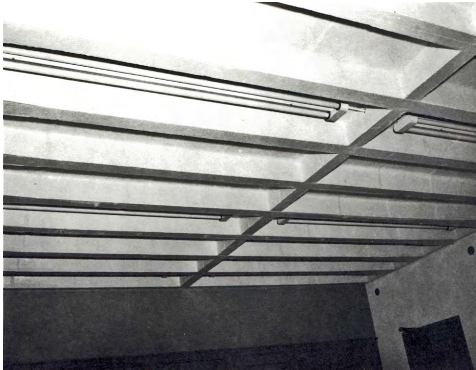
Exposed pan formed joists of Room No. 218, Ephrata Office Building. Reclamation Photograph No. 3130, December 17, 1951
