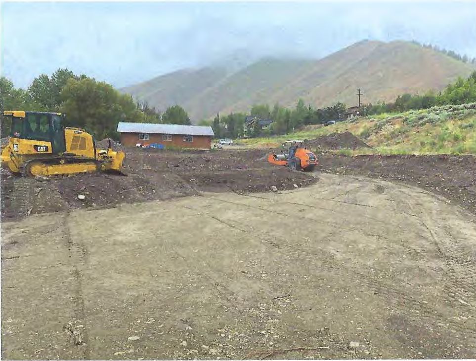
Imported sand and gravel placed in 10" loose lifts, watered and compacted with multiple passes of a vibrating smooth drum roller as structural fill. 29Jun20
