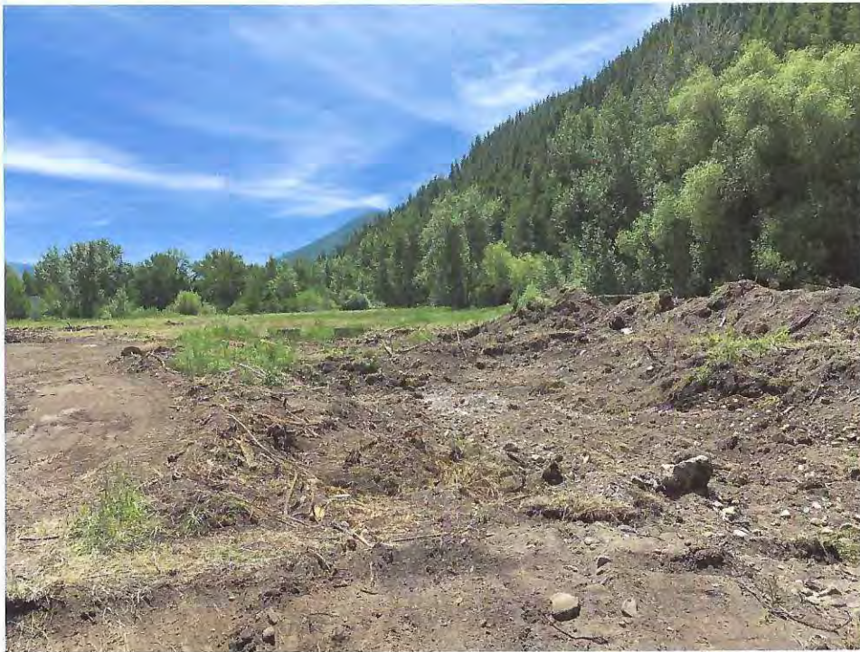
Organics, debris and disturbed soils to be removed prior to placing structural fill to match adjacent existing grade. 26Jun20
