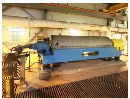
Figure 5-7. Centrifuge at Durham AWWTP in Portland, OR
