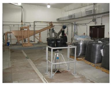
Figure 3-4. Grit chamber, conveyor, and washer room
