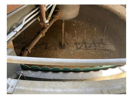
Figure 5-1. Existing gravity thickener
