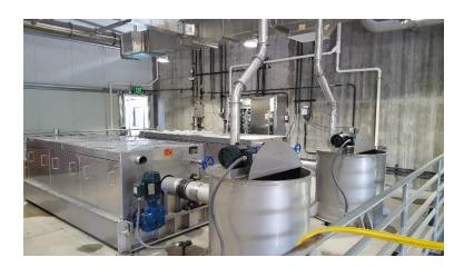
Figure 5-2. Rotary drum thickener
