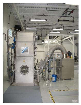
Figure 3-3. Perforated mechanical screen
