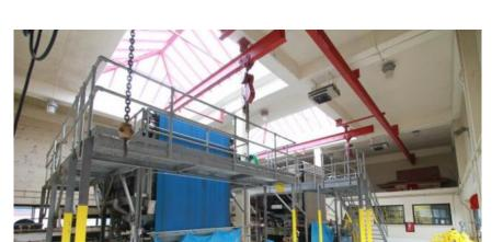
Figure 5-6. Belt filter press at the Newberg WWTP in Newberg, OR
