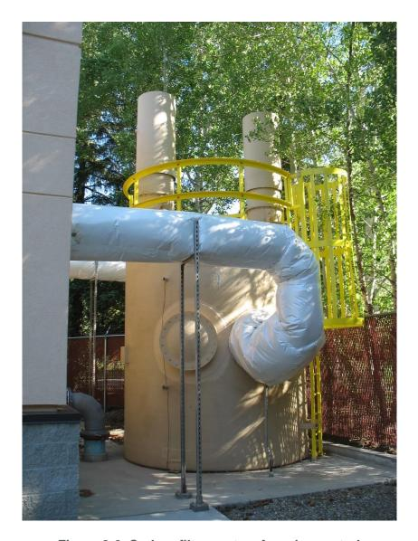
Figure 3-6. Carbon filter system for odor control
