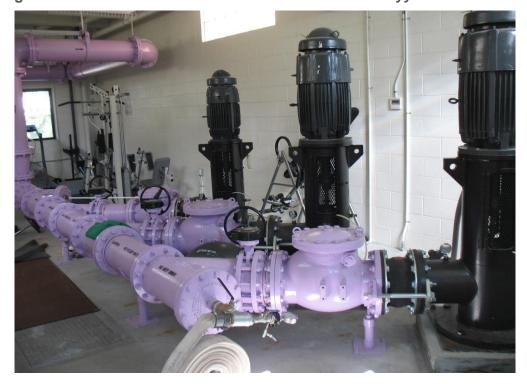
Figure 3-17. Reuse water pump room
