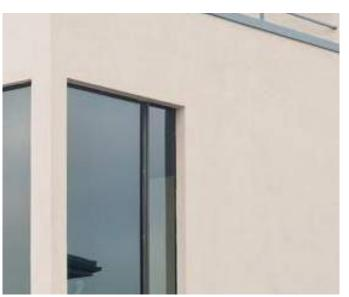
CEMENT PLASTER - 3-coat system, hard-troweled finish with 100% acrylic topcoat finish.
