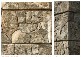
**STONE VENEER -** Montana Moss Rock natural stone dry-stack lay-up. Stainless steel masonry anchor system.
