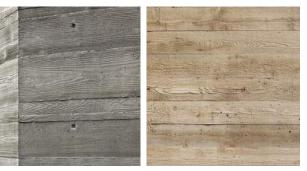
BOARD-FORMED CONCRETE - cast-in-place and stained.
