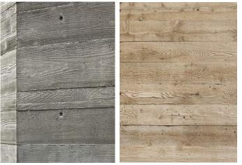
BOARD-FORMED CONCRETE - cast-in-place and stained.
