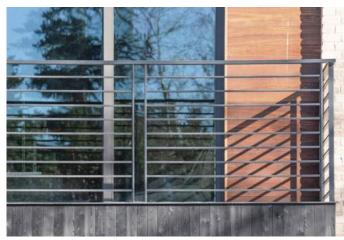
STEEL GUARD RAILINGS - galvanized and painted with WOOD TOP RAIL.
