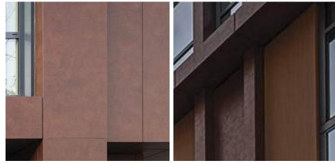
ALUMINUM PANELS with colored and textured FEVE resin-based powder coating system.
