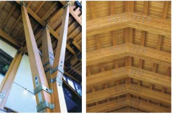
HEAVY TIMBER GLULAM BEAMS, RAFTERS AND COLUMNS with painted galvanized structural steel knife-plate connections. Fasteners to be recessed galvanized steel or stainless steel. Clear heart Western Red Cedar heavy timber purlins and T&G decking with resawn finish. Wood clear coat stain.
