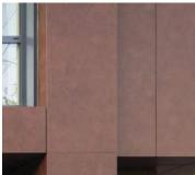
ALUMINUM PANELS with colored and textured FEVE resin-based powder coating system.
