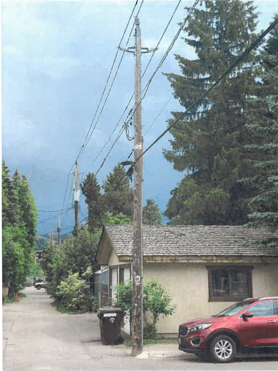
VIEW LOOKING SOUTHEAST FROM 8 TH STREET
