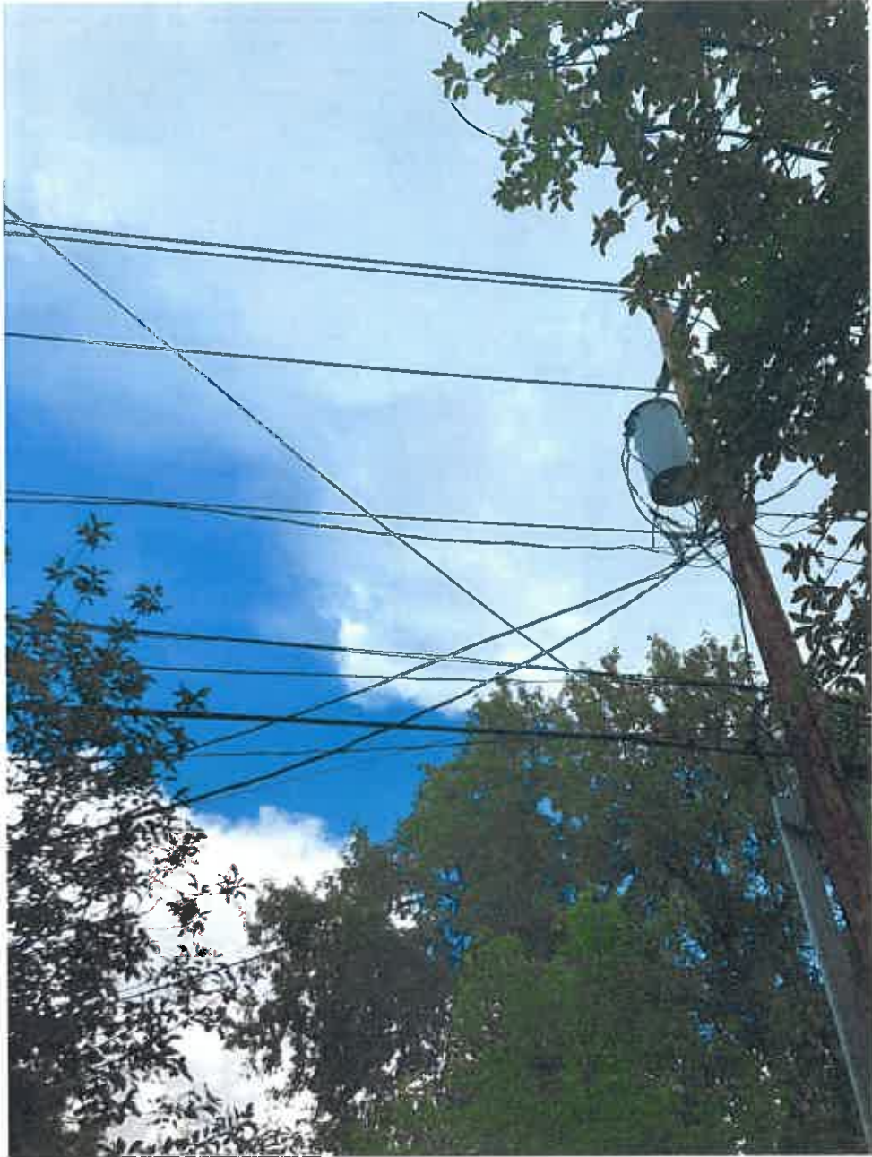
VIEW FROM LOT AT 760 WASHINGTON AVE
