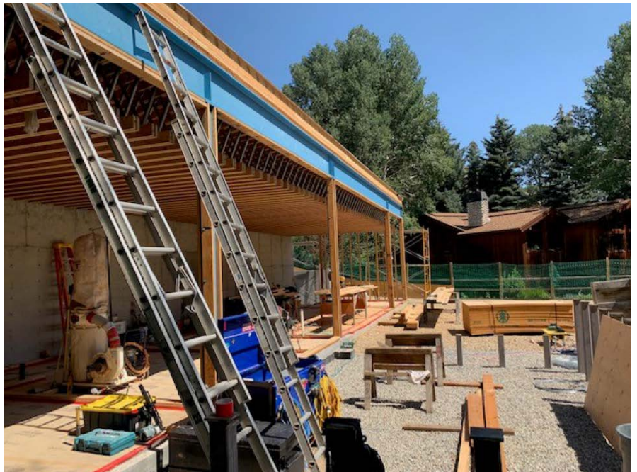
Figure 1: Picture of Project Site Taken 8/9/21
