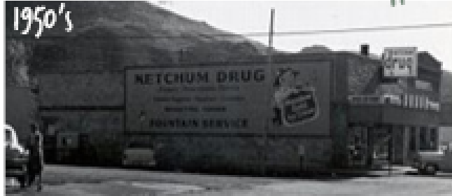
Windermere Real Estate Office
