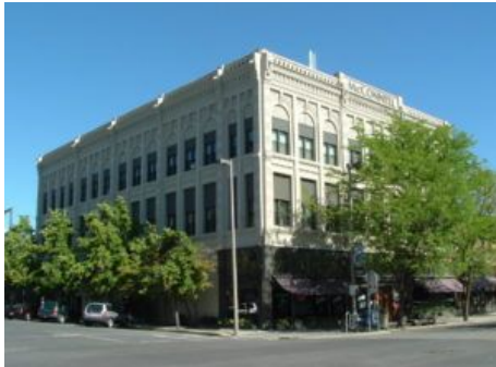
McConnell Building, Moscow ($175K) 1984 Source: Idaho State Historical Society
