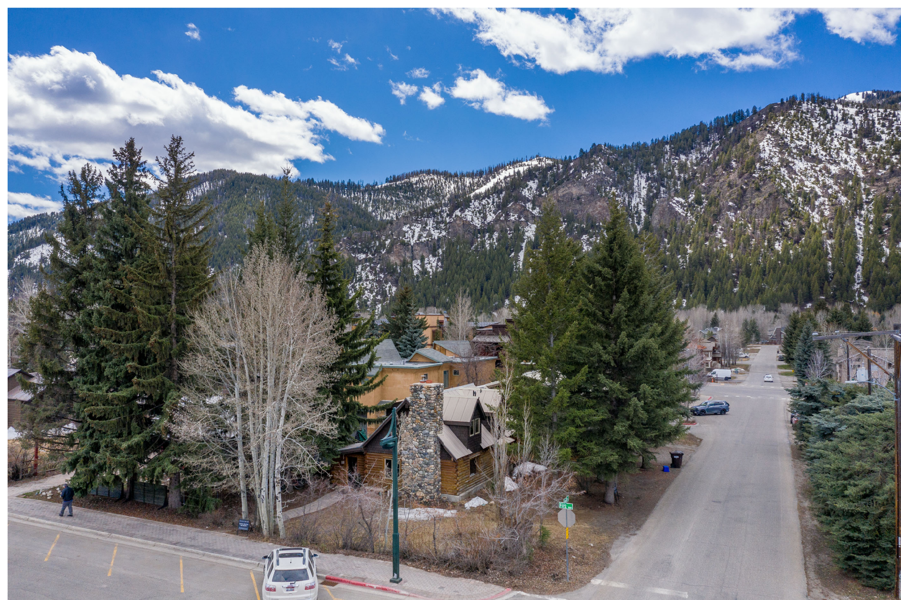
BIRDS EYE VIEW OF SITE LOOKING SOUTH WEST
