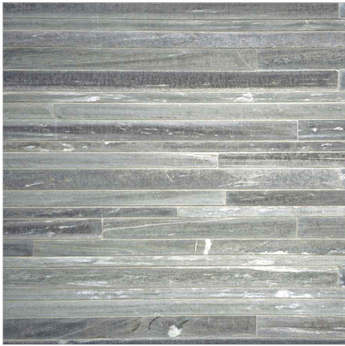
3) Stone Cladding At exterior walls
