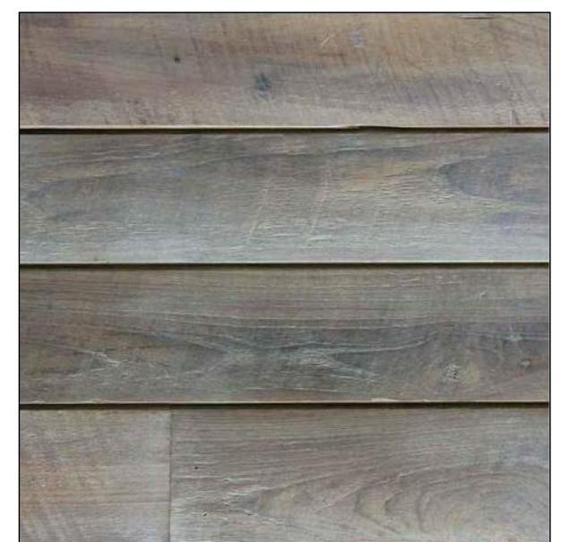
Typical Wood Siding Rustic reclaimed fir siding
