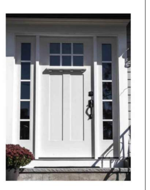
Typical Trim Accents White painted roof fascia, misc. painted trims
