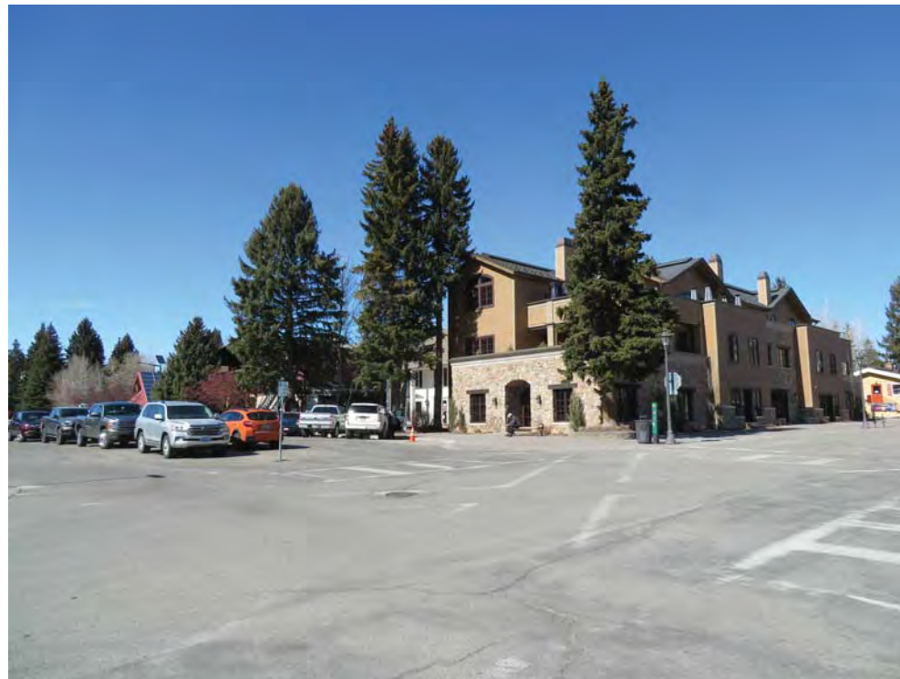
SW CORNER, EAST AVE. & 4TH ST.
