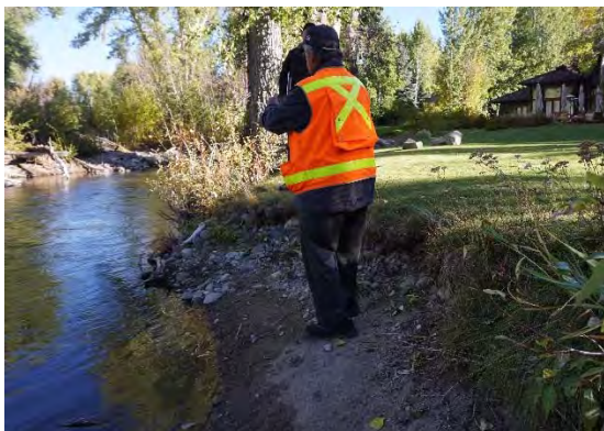
Figure 1: Eroding channel bank in project transition area.
