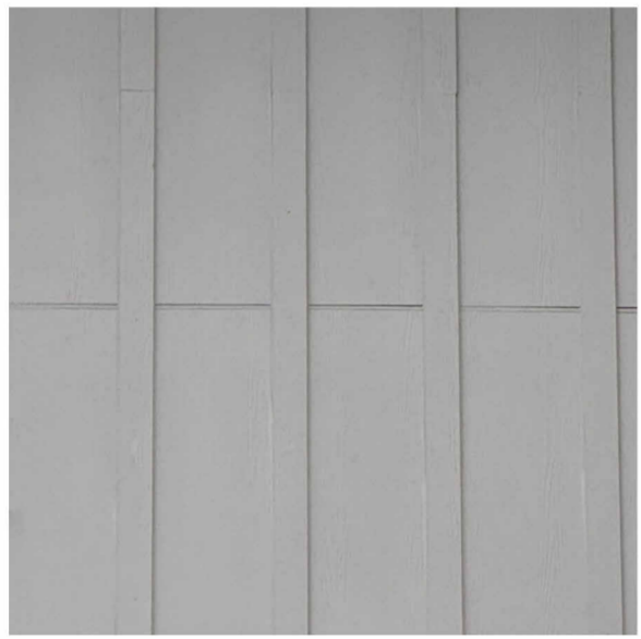
BOARD AND BATTEN SIDING TO MATCH EXISTING
