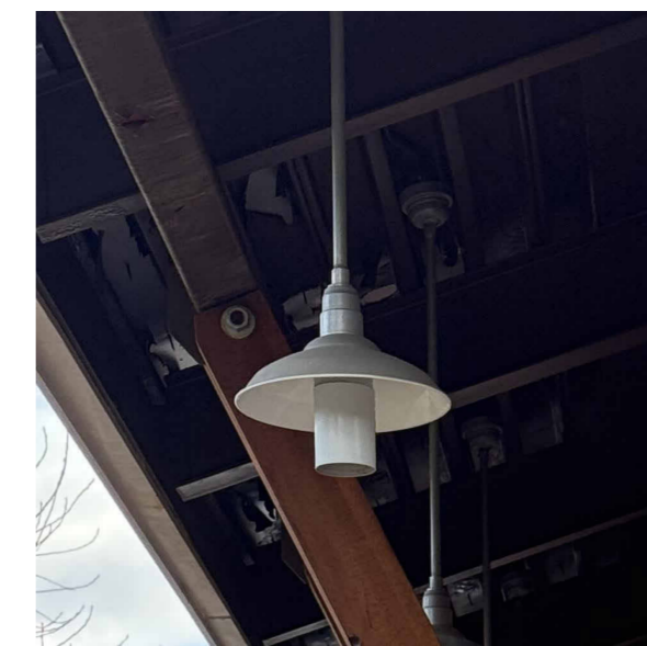
E2 PENDANT FULL CUT-OFF 2700K 9W LED - 800 lm ±
