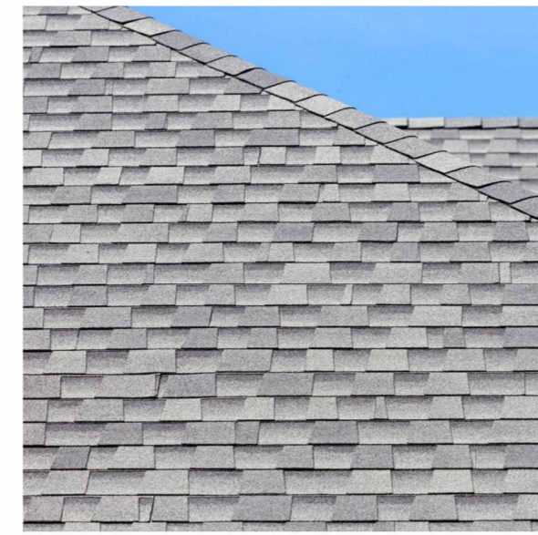
SHINGLE SLOPED ROOFING FINISH TO MATCH EXISTING
