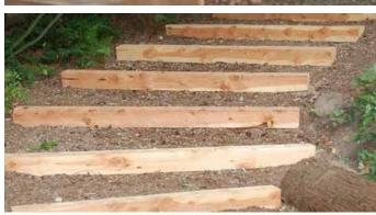
Natural timber steps set into the hillside with steel braces
