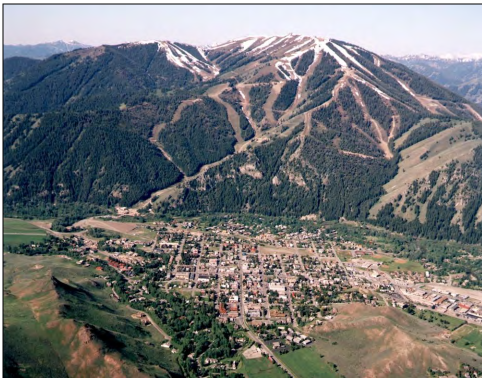
Figure 20. Aerial view of Bald Mountain, view southwest.
