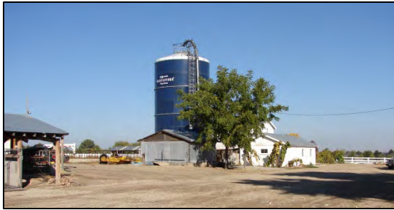
Silos like this one, constructed of fiberglass and metal, were a post-World War II innovation in silo construction. Photo by TAG.
