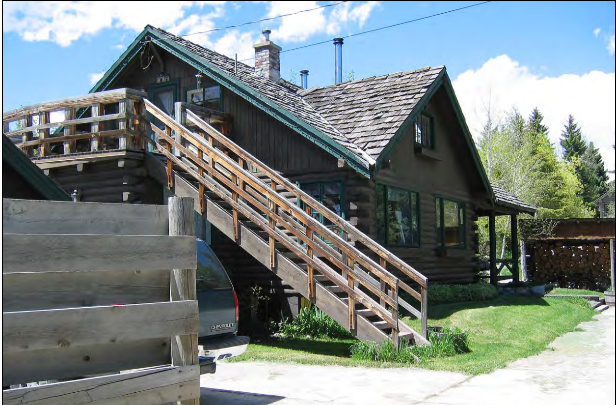
Figure 4. Fuller House at 90 Meadow Circle was a typical house built at Mortgage Row in 1948. Digital Image MR 13 # 13, view northwest.
