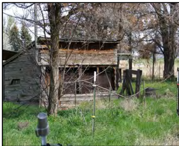
No longer used, this chicken coop is one of several buildings left at a small farmstead on Lamont Road. Photo by TAG.
