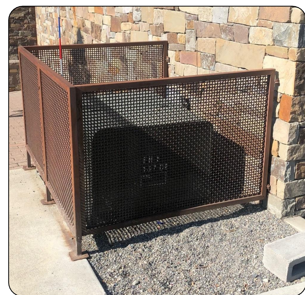
PHOTO: TRANSFORMER COVER EXAMPLE
