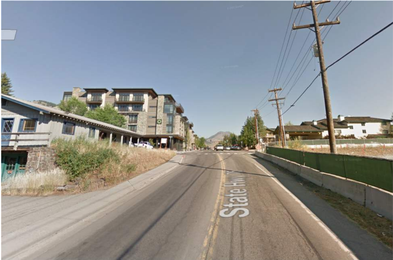
Figure 12. River Street Intersection View from the South.
