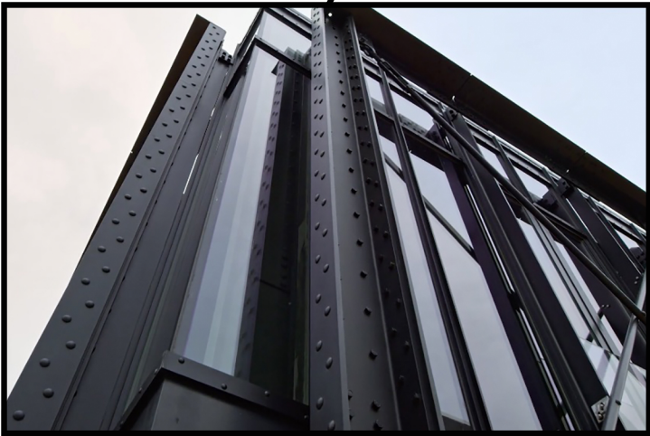
PAINTED METAL FACADE
