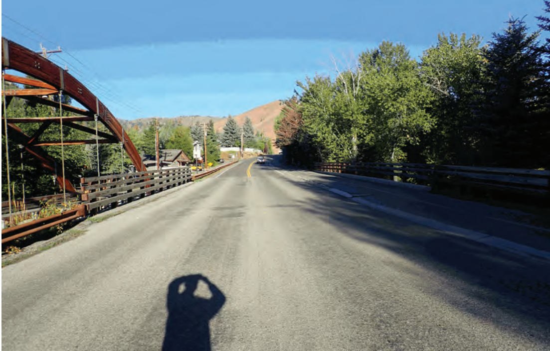
Approach looking west.
