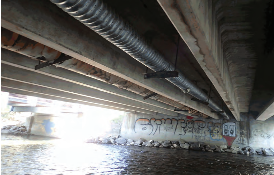
Underside and west abutment looking southwest.
