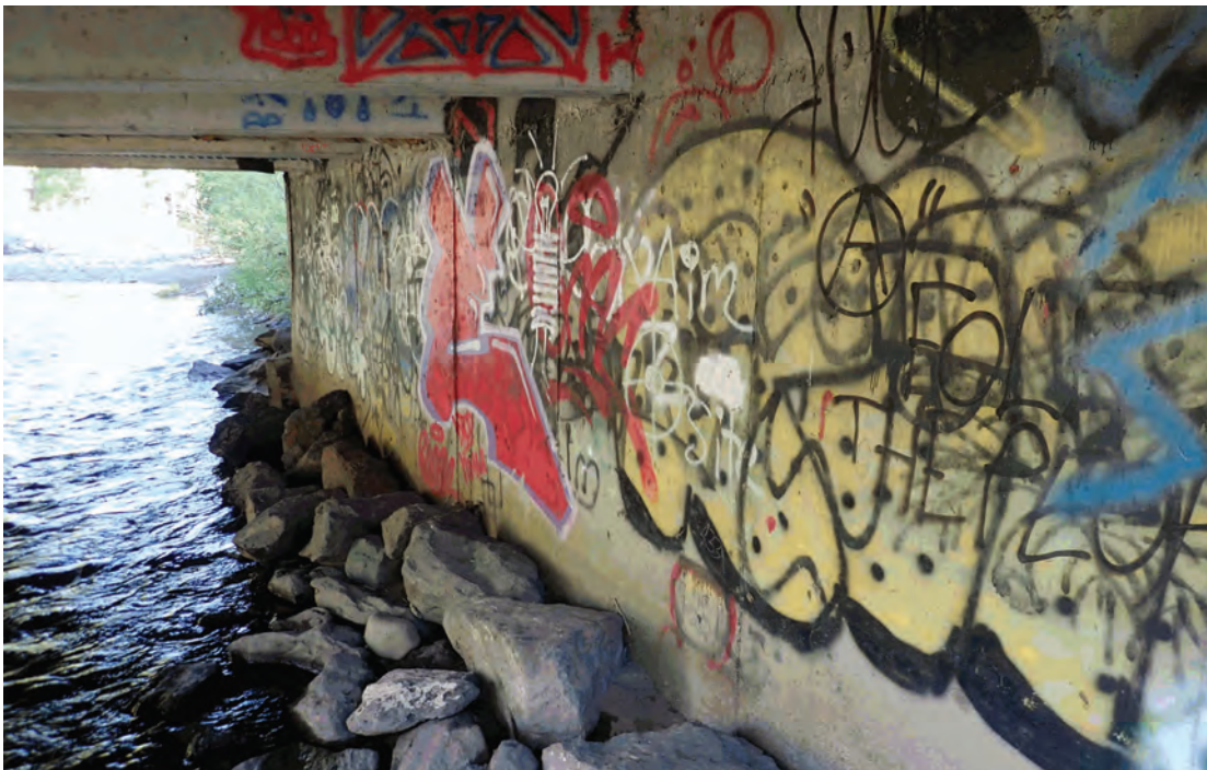
East abutment looking northeast.
