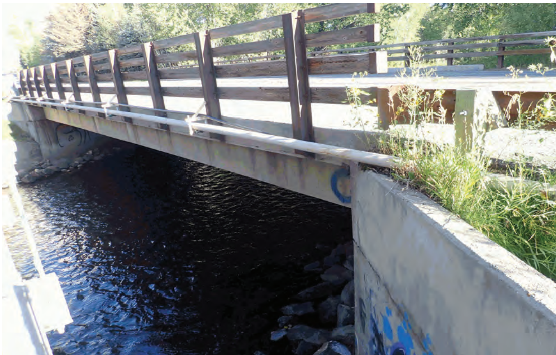
Overall looking northwest.
