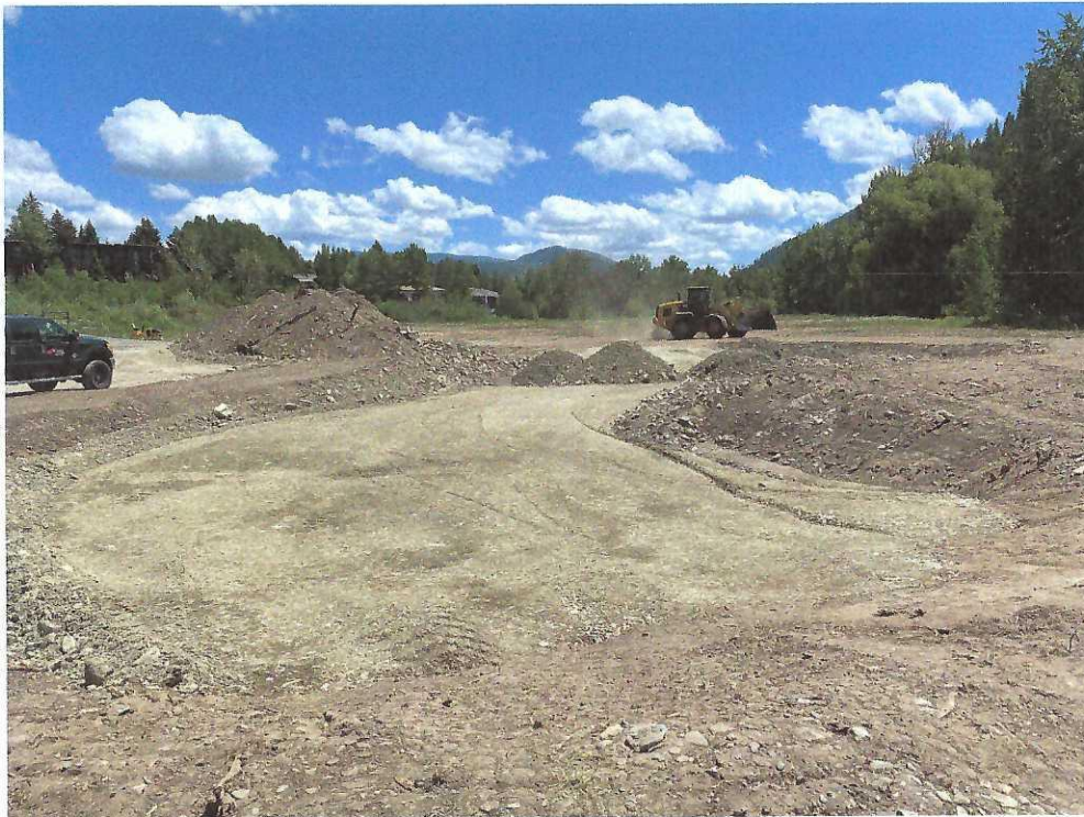
Up to 5 feet of imported sand and gravel placed to match adjacent existing grade. 1Jul20
