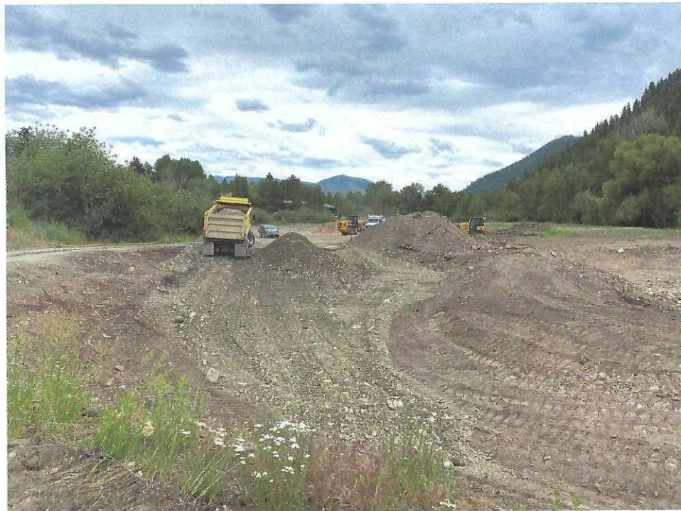
Imported sand and gravel being placed on compacted and approved native sand and gravel subgrade. 27Jun20
