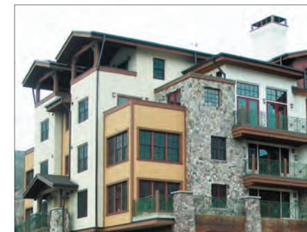
A flat roof may be used as an accent to break up the perceived mass of the overall building
