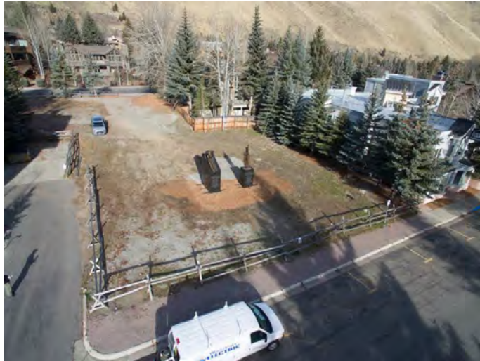
Birds eye view looking at SW corner of project lot, gentle slope from Howard Drive to Picabo.
