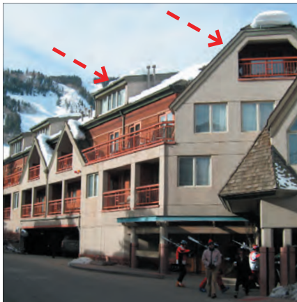
Place top floors within the roof form to reduce the perceived height of a building.
