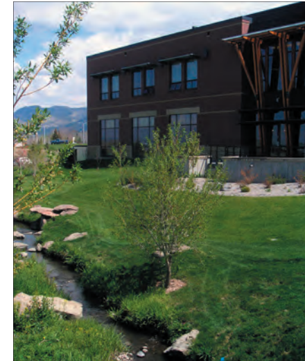
Use open drainage swales with natural linings, native rocks and other local materials.
