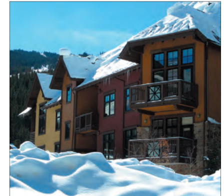
Variations in wall planes and architectural detailing help to minimize the perceived scale of the building.
