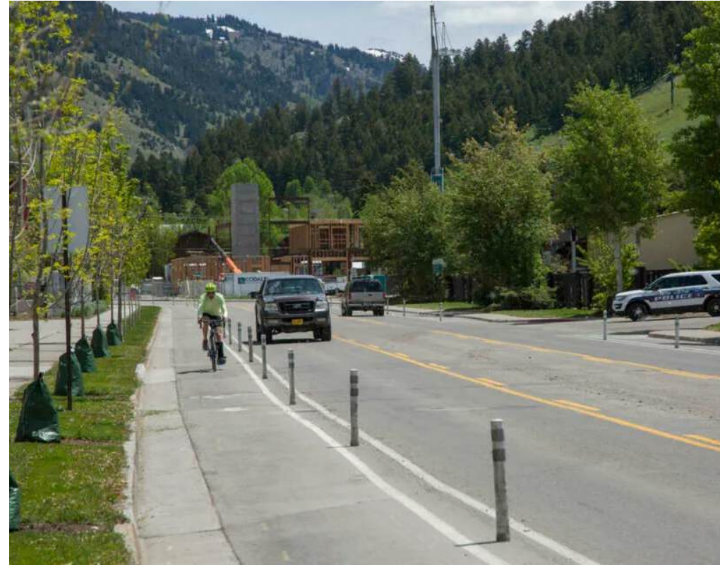
BUFFERED bike lane at street level Snow King Ave | Jackson, WY
