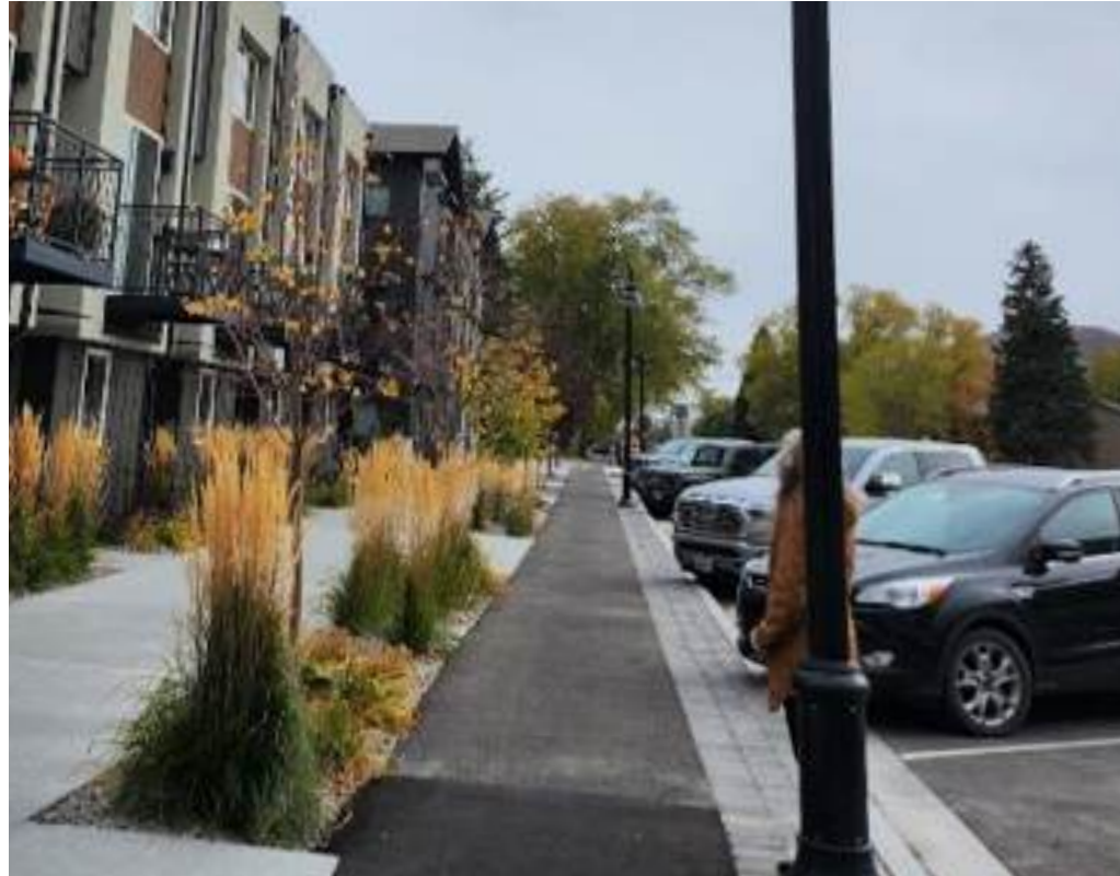
PROTECTED bike lane at sidewalk level River St | Hailey, ID
