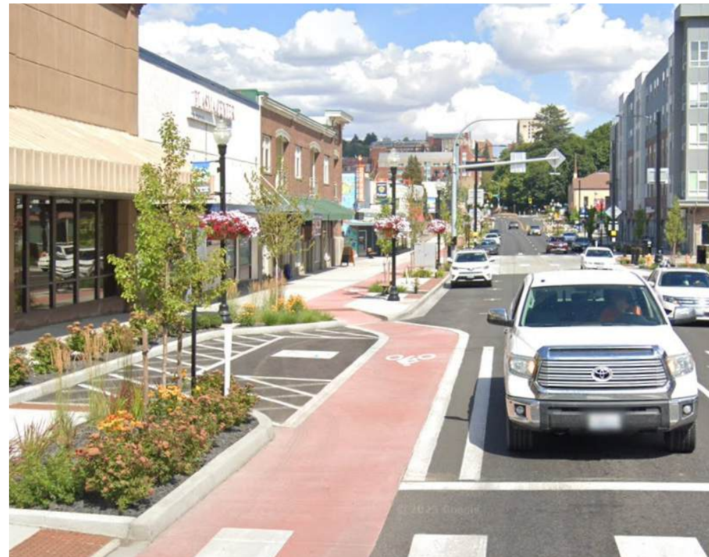
PROTECTED bike lane at sidewalk level transitioning to street level at intersection Main St | Pullman, WA
