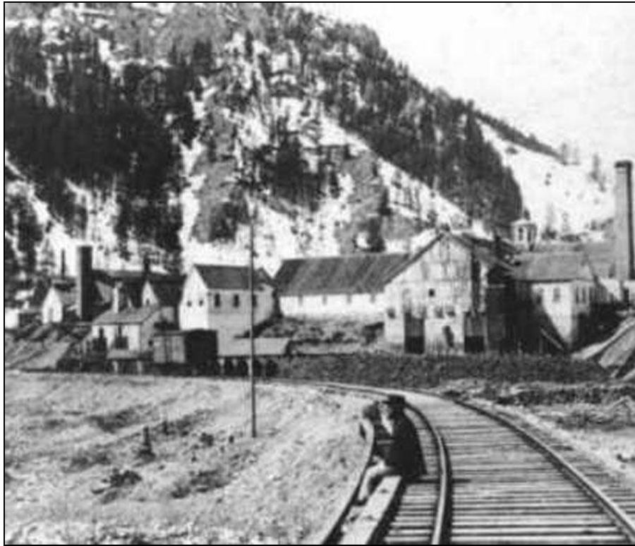
Figure 17b. Philadelphia Smelter and Oregon Short Line Railroad courtesy Regional History Department of the Community Library, Ketchum.
