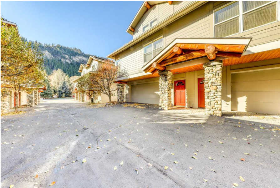
Townhome with fire sprinklers
