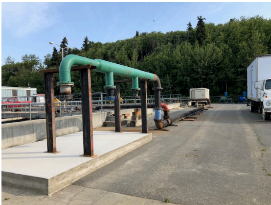
Temp Blower Pad and Piping
