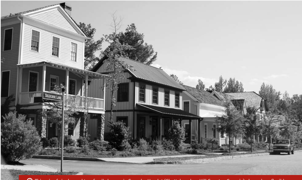
➡ This mix of single- and two-family homes in Serenbe Hamlet (Chattahoochee Hill Country, Georgia) shows how flexible standards can encourage high-quality design.
