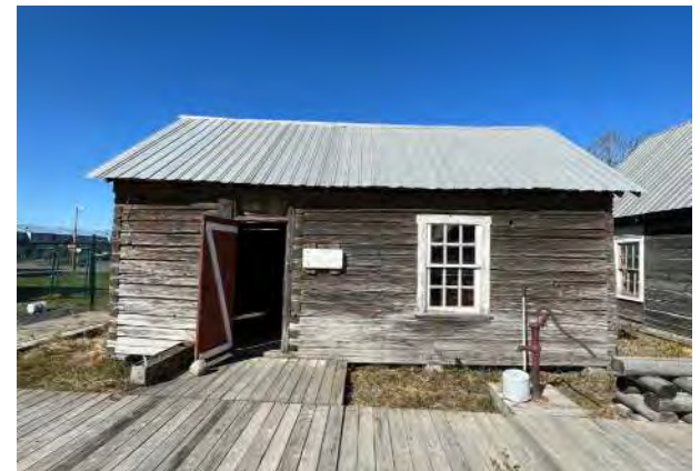
Kenai Historic Cabin Park
