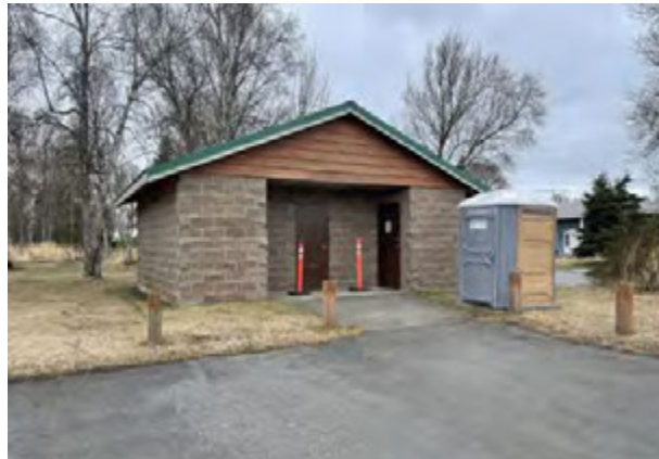
Seasonal bathroom structure and portable toilet
