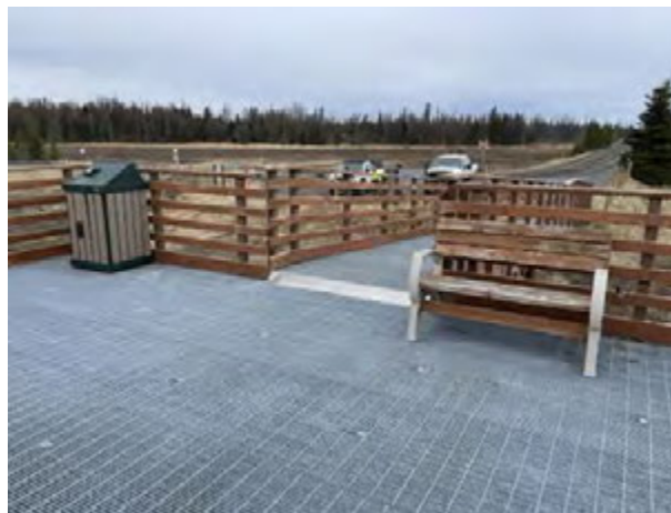
Bench and waste receptacle on platform
