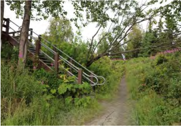
Stair access from the boardwalk to the riverbank
