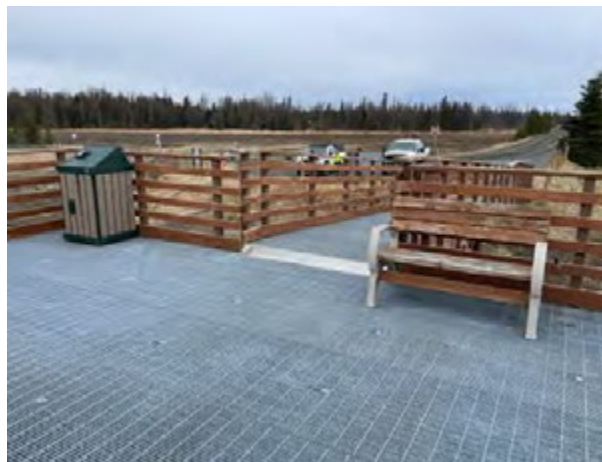
Bench and waste receptacle on platform
