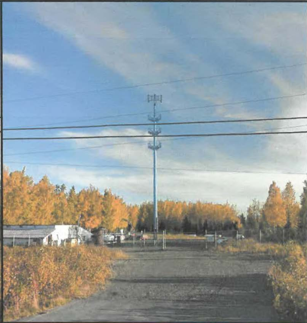
After - Looking North
