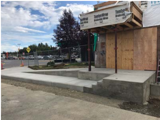
North End New Ramp/Stairs
