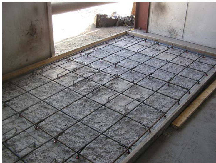
New Blower Pad prepped for concrete
